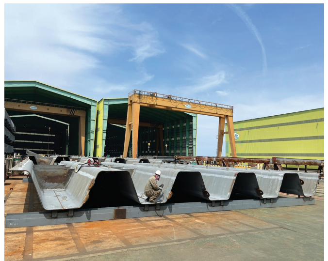
BEACHHEAD FOR METHANOL TANK
